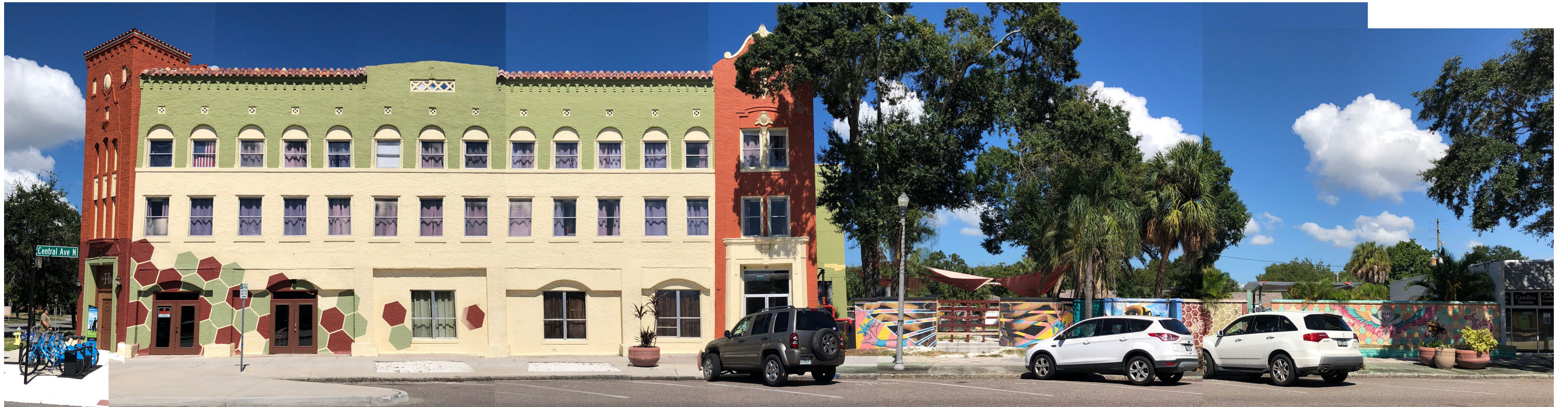
SOUTH ELEVATION (CENTRAL AVENUE)
