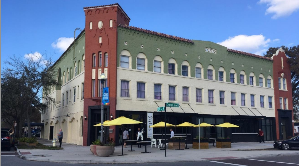
Figure 2: Image of recently installed storefronts.
