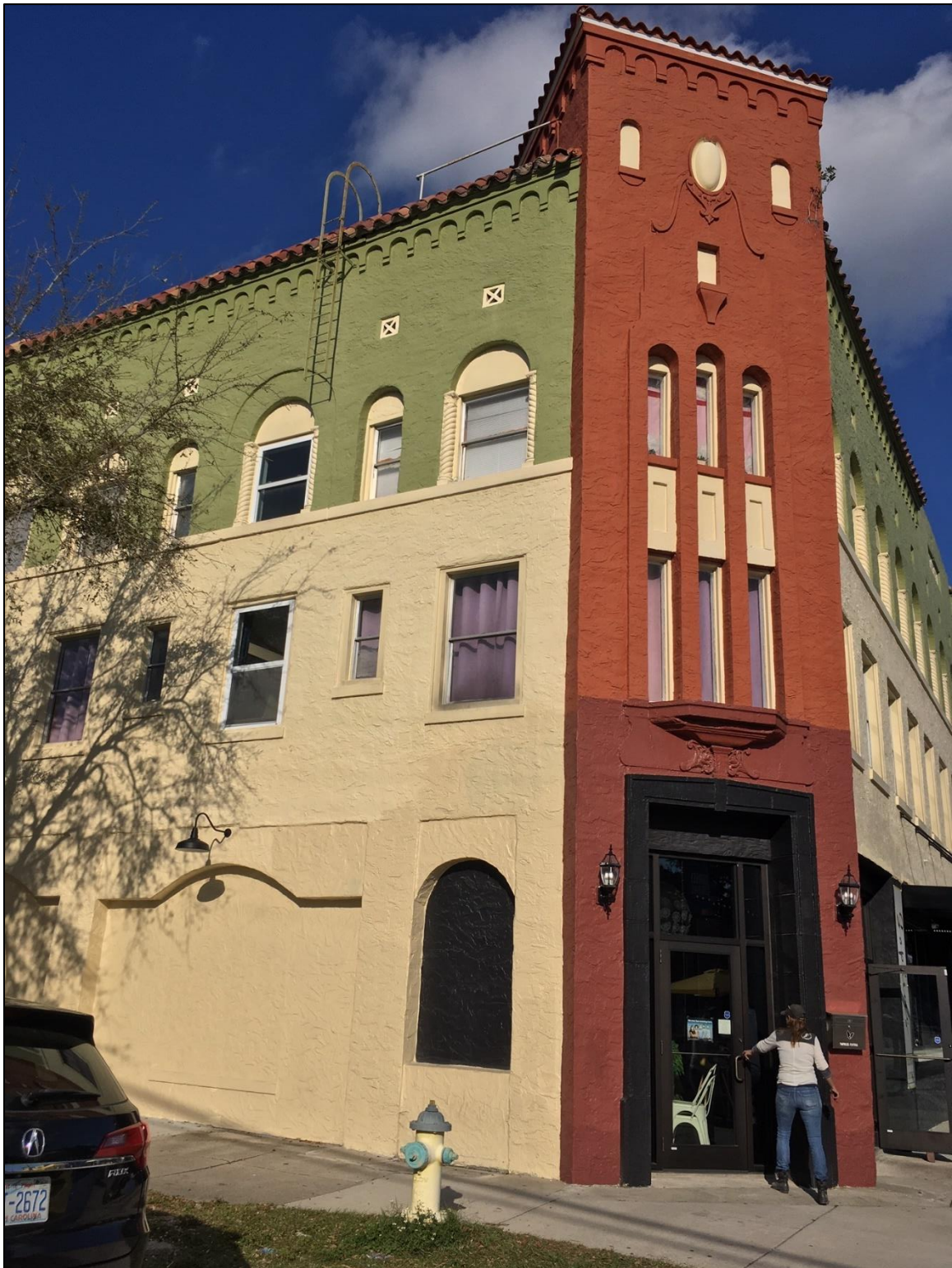
Figure 4: Photograph shows two windows that have been replaced with modern white windows, which are similar to the proposed windows.
